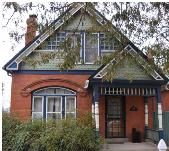
4. Queen Anne cottage. Note the decorative fish scale shingles and barge boards in the forward facing gable, the spindle columns and fretwork on the projecting front porch, the arched windows on the first floor with decorative jack arch and corbels.
