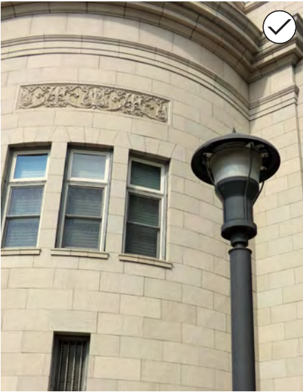
128. Use low, shielded, fixtures with down-lighting, or light bollards within landscaping to illuminate pedestrian walkways if needed.
