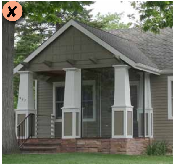
Figure 162: This porch is not in proportion with the historic context since the porch columns are oversized.
