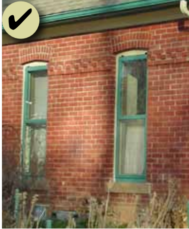
Figure 81: Repair and weatherization is often more energy efficient, and less expensive, than replacement.
