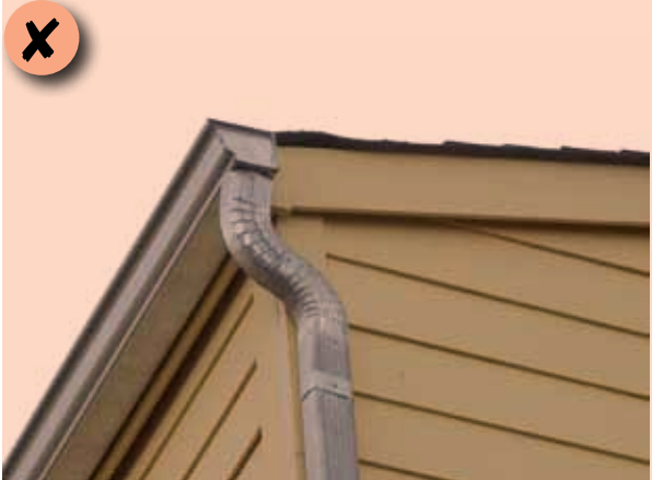
Figure 175: This eave is inappropriate since it does not provide an overhang.
