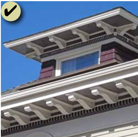
Figure 64: Maintain significant character-defining features, including: projecting cornices, decorative moldings and brackets and dentils and shingle siding at dormer.
