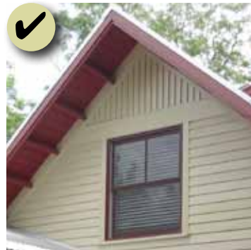
Figure 174: This combination of horizontal and vertical wood siding is an appropriate application. Note how the vertical boards highlight the gable end in a unique design approach.
