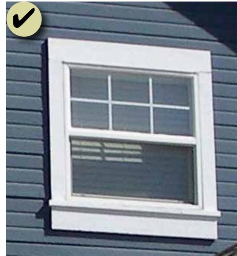
Figure 169: Set back a window or door from the outside wall plane so a reveal is evident, resulting in a shadow line around the opening. The window or door should not appear flush with the outside wall plane.
