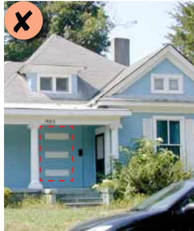
Figure 85: This three pane window alteration is inappropriate and should be restored to its original historic configuration.
