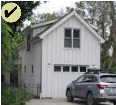
Figure 188: This new compatible accessory building with a living unit above provides similar materials found on other historic accessory buildings.
