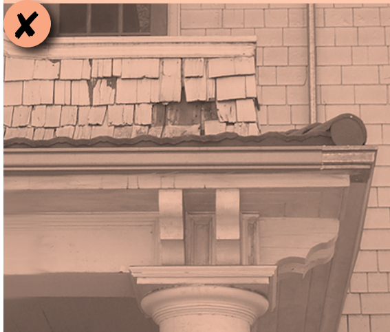
Figure 69: Do not remove damaged materials that can be repaired. In this case, loose shingles may be re-secured while missing ones may be replaced.
