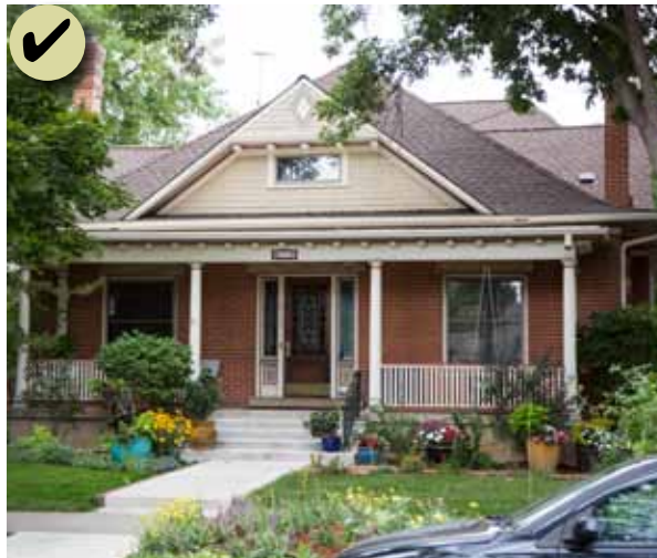
Figure 61: One-story cottage homes are a common style throughout the Old Town Neighborhoods Character Areas.
