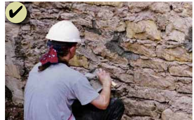
Figure 116: Re-point historic masonry foundations to match the historic design.
