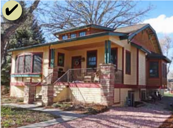
Figure 110: Clipped, side-gable roof form with loft dormer
