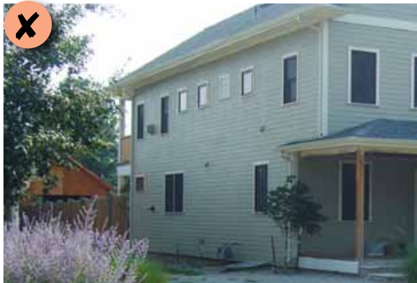
Figure 154: This building wall is inappropriate; it is too long and does not have any wall offsets.
