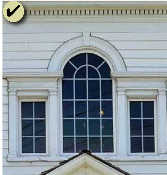
Figure 65: This palladian window with wood tracery is a character-defining feature that helps to convey the architectural style and should be preserved.
