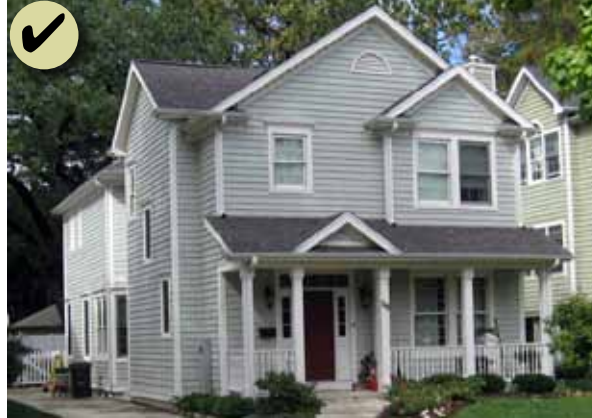
Figure 142: This building has several compatible features such as the traditional massing, porch, articulation and materiality.
