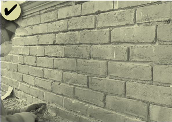
Figure 76: Re-point mortar joints where there is evidence of deterioration. This shall match the historic design.
