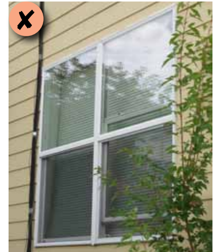
Figure 170: A window should not appear flush with the outside wall plane.
