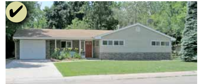
Figure 130: Traditionally, most parking was accessed from alleys in the neighborhoods; however, Character Area 6 reflects a development pattern where much of the parking access is off of the street leading to an attached garage.
