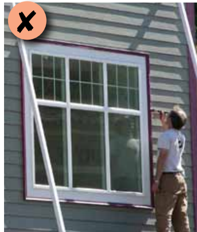
Figure 86: The windows and siding have both been inappropriately replaced with vinyl.
