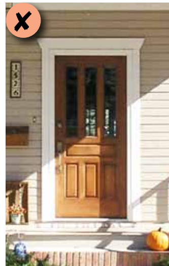
Figure 97: This three-pane replacement door is not typical for most of the historic styles located within the neighborhoods. A simple single-pane window door should be used.
