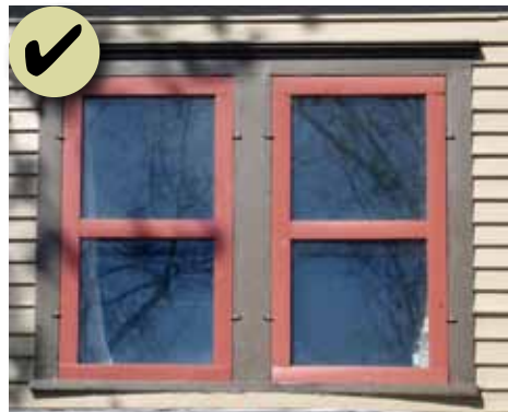
Figure 92: The storm windows match the opening; however, it would be more appropriate if the frames matched the historic window sash similar to the image shown above.
