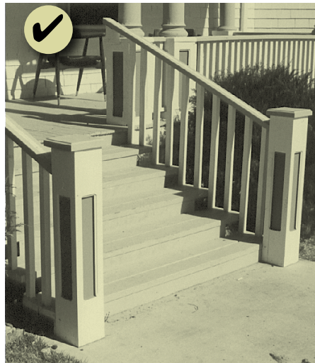
Figure 72: After: Railing has been repaired and the base of the post has been replaced in-kind. This is an appropriate approach.
