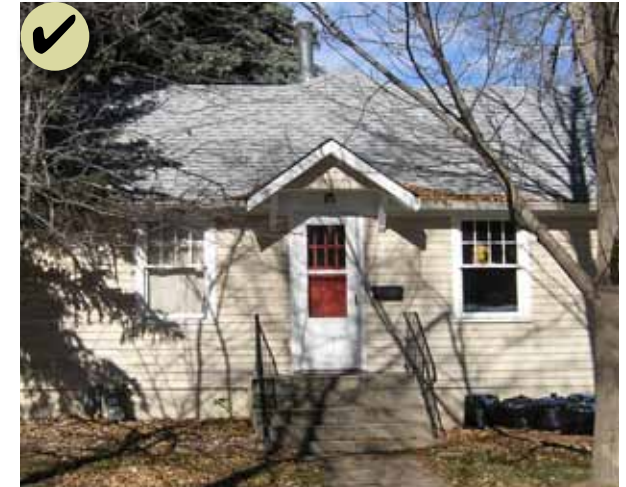
Figure 60: One-story, cross gable roof Minimal Traditional residence.
