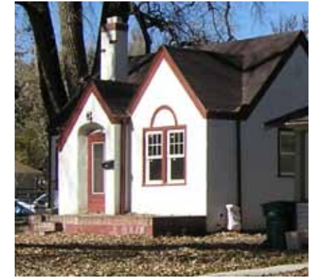
Figure 29: Character Area 3 with hints of Tudor building form
