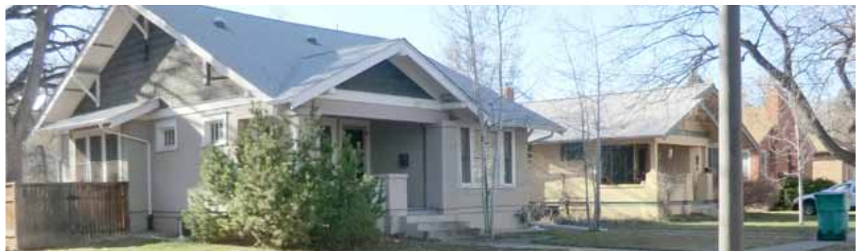
Figure 39: Character Area 4 Craftsman in the foreground has been appropriately rehabilitated. Note the retention of building fabric and detailing.
