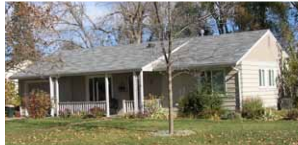
Figure 53: Character Area 6 Ranch with porch front addition
