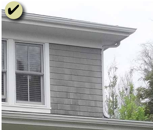
Figure 178: Boxed eaves with generous overhangs are appropriate.
