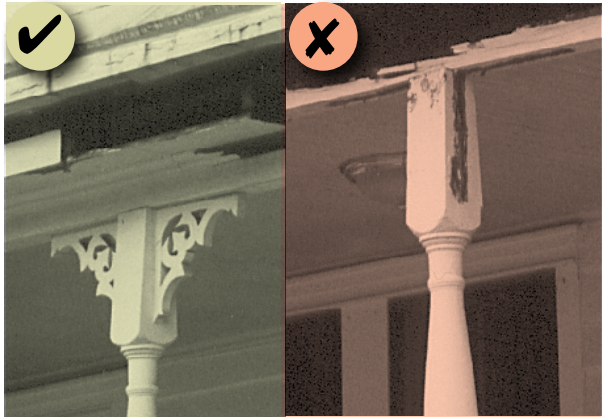
Figure 73: Replace missing original details in kind.
