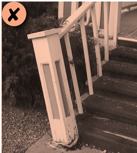
Figure 71: Before: A deteriorated railing should be repaired not replaced when feasible.
