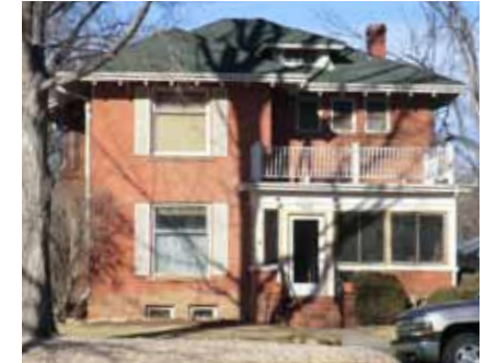
Figure 9: Character Area I Vernacular with an altered porch and Craftsman detailing at the eave
