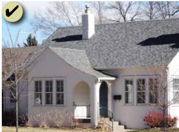
Figure 113: Gable roof with shallow eave over the primary form and a splayed gable roof form tops the one-story projecting entry feature.
